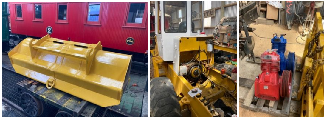
Bucket attachments welded and painted.
