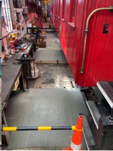
Raised concrete floor sections
