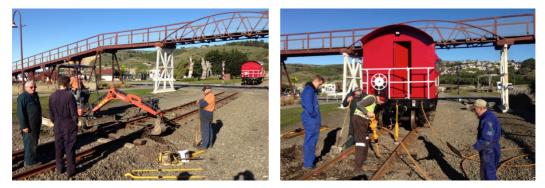
A hired backhoe dug out old sleepers, replacing them with larger concrete ones. These were lifted, and attached to the rails with Pandrol clips. Ballast was tamped under the track using air tools driven from the CW's compressor - less physically stressful than the heavy old 'Wacker' petrol-powered bone-shaker.
